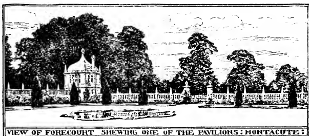
VIEW OF FORECOURT SHEWING ONE OF THE PAVILIONS: MONTACUTE:
